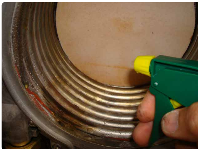
Figure 150 Cleaning the heat exchanger
