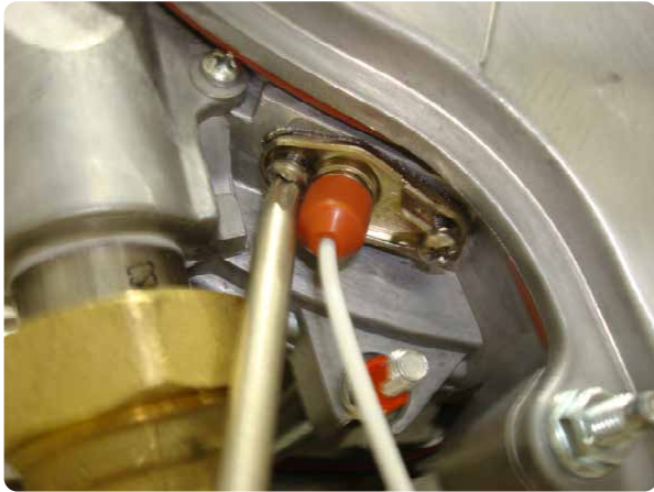
Figure 142 Removal of Ignition electrode
