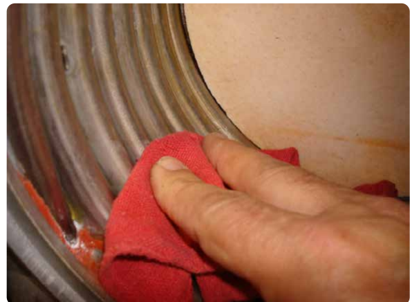
Figure 152 Cleaning the heat exchanger
