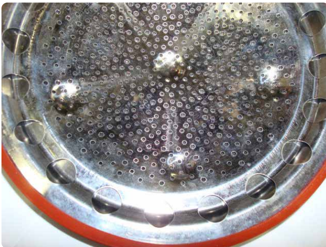
Figure 147 Inspecting interior and cleaning the burner
