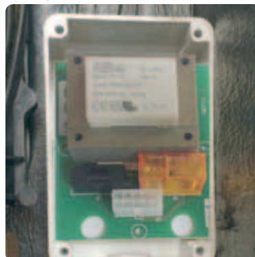
Figure 67 Thermostat-Relay box terminals Combi and Central Heating boilers
