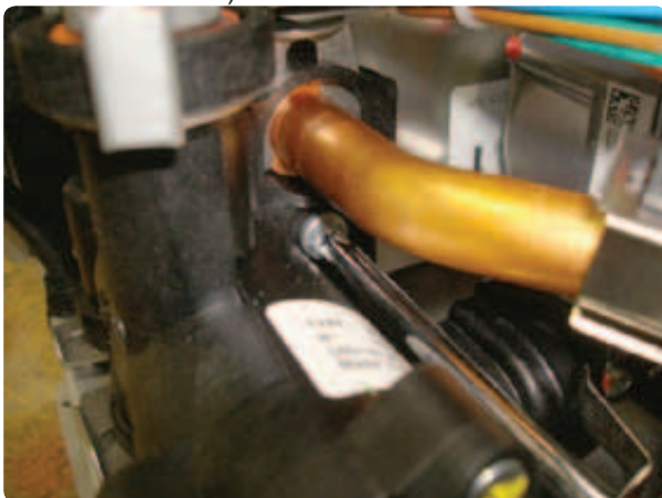
Figure 157 Removal of flat plate heat exchanger (screw on left side) (Combi Only 80/120 shown)
