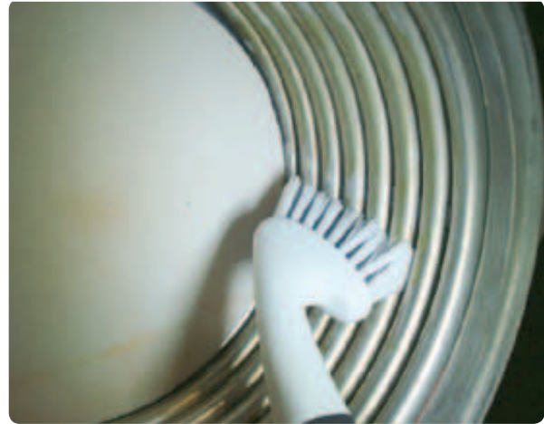
Figure 151 Cleaning the heat exchanger
