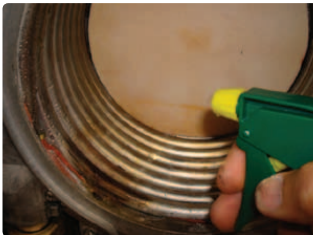
Figure 150 Cleaning the heat exchanger
