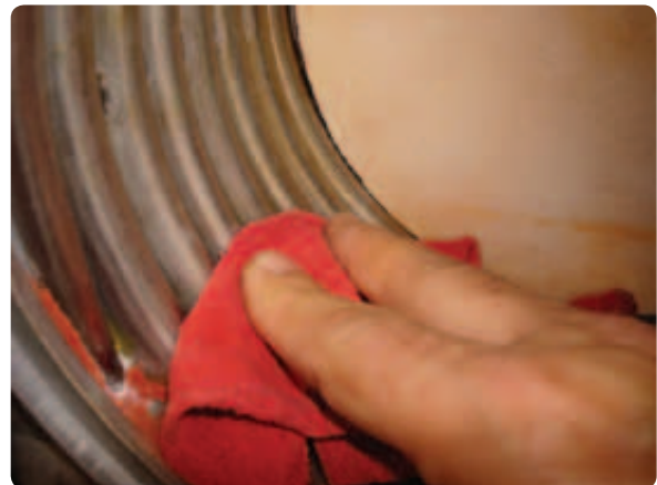
Figure 152 Cleaning the heat exchanger
